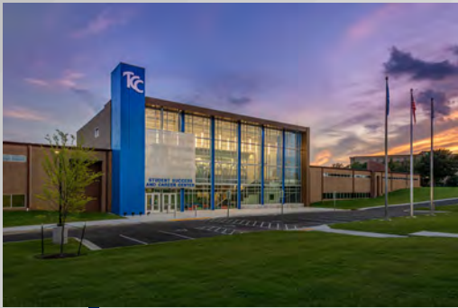
Southeast Campus SSC Completed August 2019
